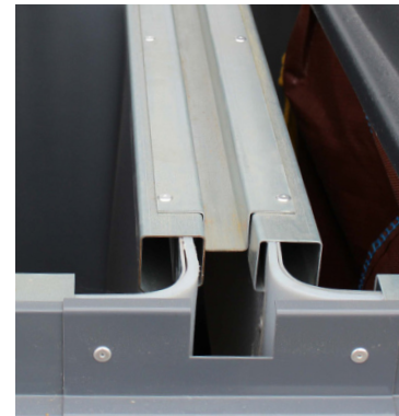
Image 3. Attaching the U-profile strip
