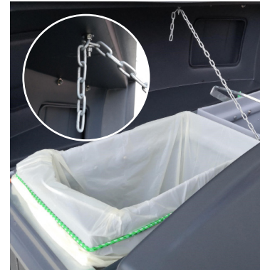
Image 6. Installation of the side hinge chain and disposable bag
